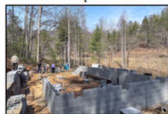
Ruth's Refuge (staff duplex) in progress
